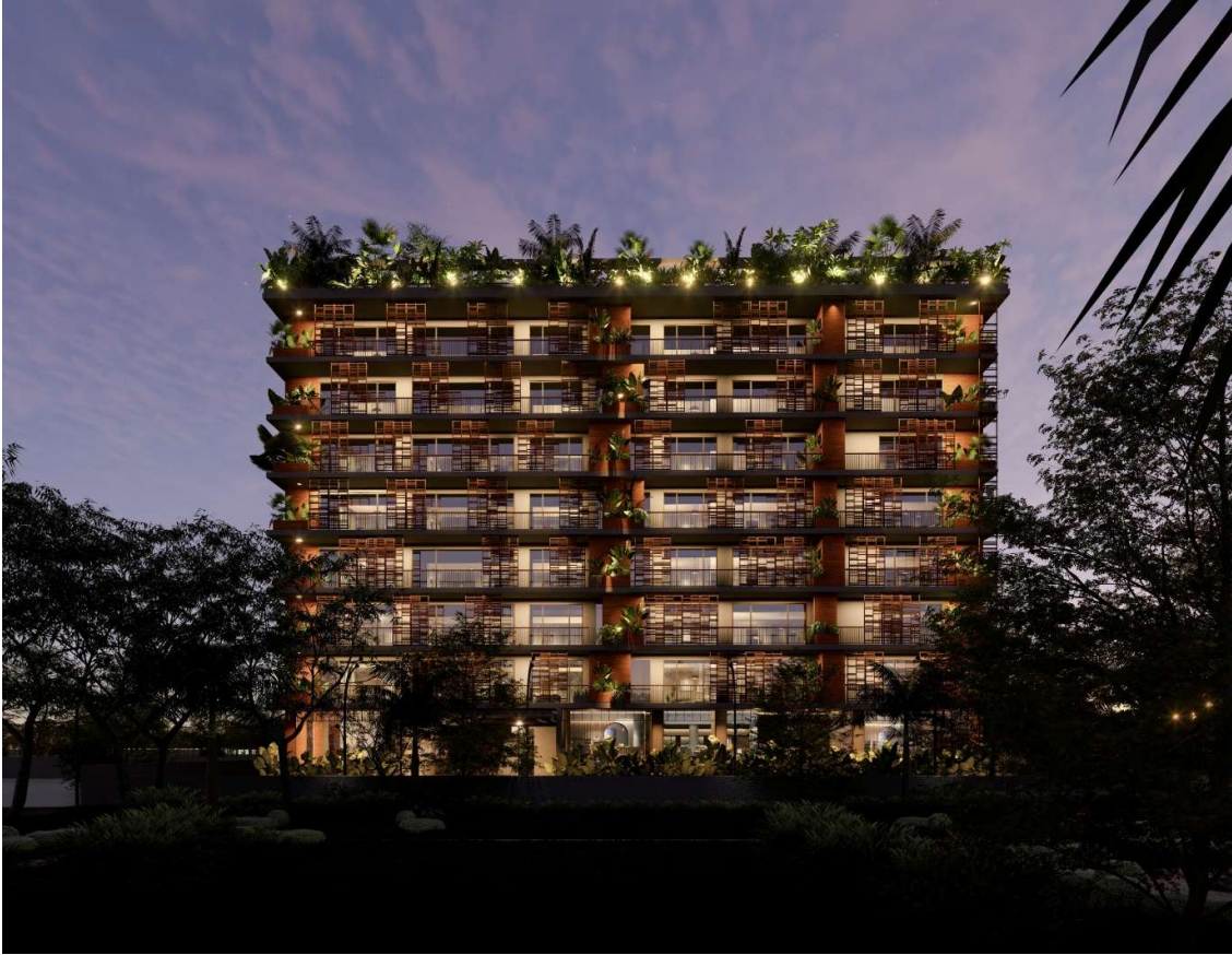
5. Margao – G + 8 Story buildings having 24 apartments of 3000 Sft each
